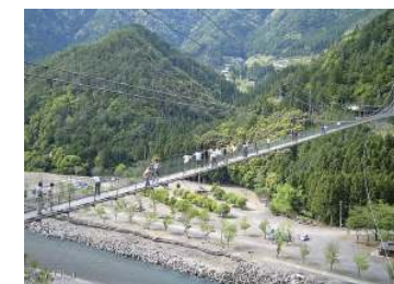
Suspension Bridge of Tanise (Nara)
